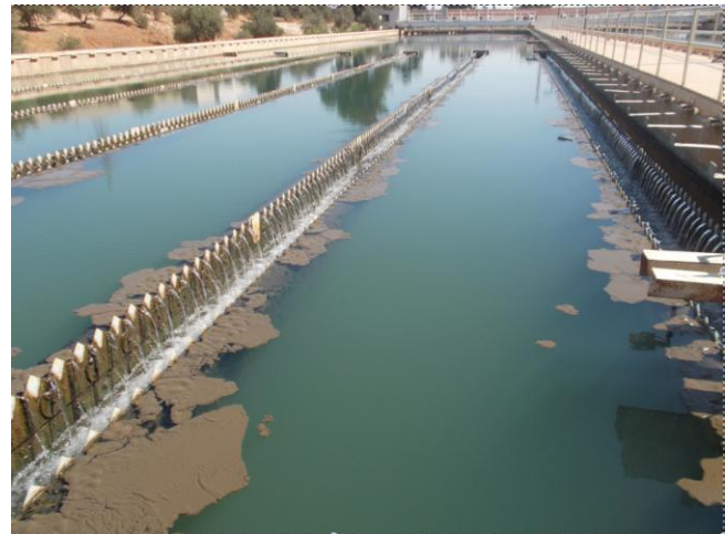
Figure 2: Sedimentation Basins at Zai Water Treatment Plant
